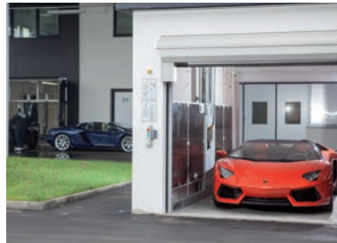
Both elevator systems serve the two floors of the building for the movement of cars during the phases of assembly.
