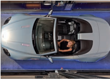
The system has two lateral columns and is suitable for height differences up to 11.9 m with a minimum shaft of 80 cm and an invisible arch beneath the platform.
