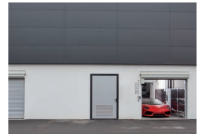
The car lift closures have been supplied by the company Hörmann. They consist of 6 extremely quiet and fast rolling shutters.
