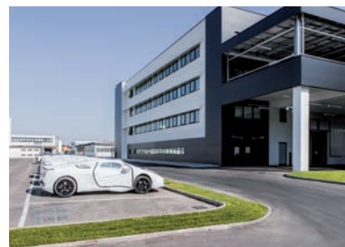
Special 3m x 1m laminated stoneware plates in "Lamborghini Black" were laid horizontally with an exposed anchoring system.
