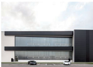
The facade of the new Protoshop of Lamborghini is in part created with a system of ventilated walls to satisfy all thermal and acoustical requirements.
