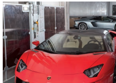
The car lift can be controlled through a push-button panel and a magnetic card.
