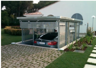
This car lift rise is 270 cm. In this installation, 2 parking spaces were obtained, one on the platform and one in the basement.
