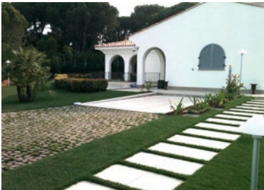
The covering roof of the car lift is at the same level of the courtyard/garden and is crossable. Cars with an overall weight of 3,000 kg can be parked.
